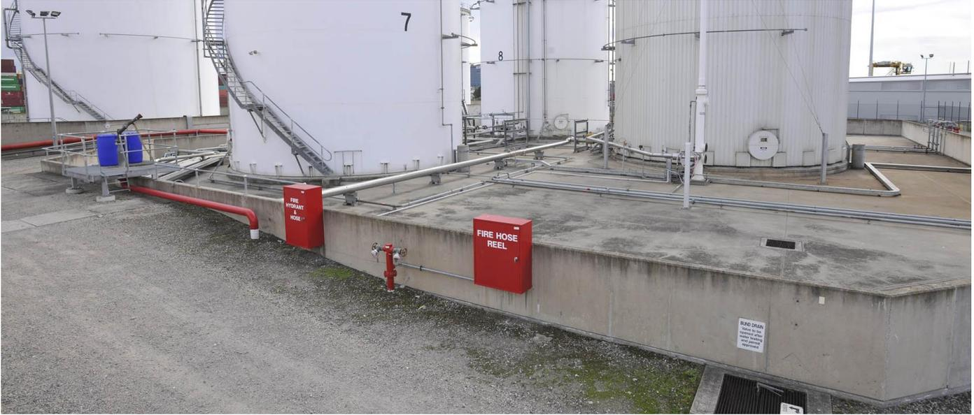
Figure 5: Image of an industry site that uses bunding around their tanks as secondary containment.
