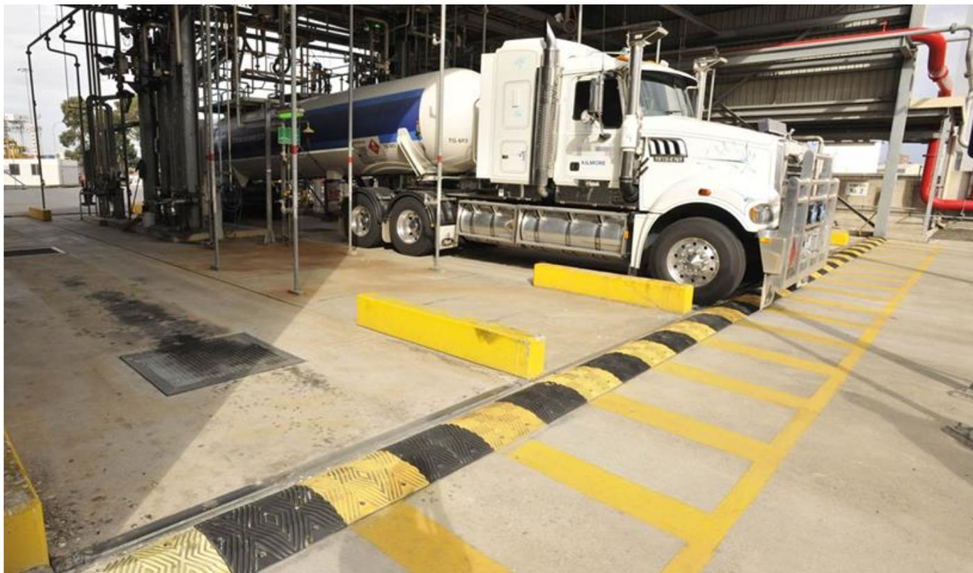
Figure 14: Rollover bunds can be a useful form of containment that can prevent liquids from leaving the work area.
